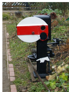
The repainted and refurbished Ground Signal ready for operation again.
