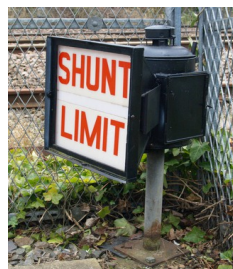
The rebuilt Shunt Limit sign back in position following its spontaneous combustion.
