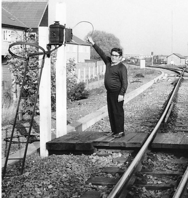
**Chesterton Junction, Cambridge was where the St Ives branch left the main line. The Signalman is placing the hoop and pouch containing the single line token into the holder for collection by the driver. The lamp illuminates the hoop at night. These items are now on display in the 'box garden, donated by Andy Buckley who took the photo prior to closure in 1980s. Below Tony Furse re-enacts the scene. New posts have been erected but the rest is as shown in the top shot.**
